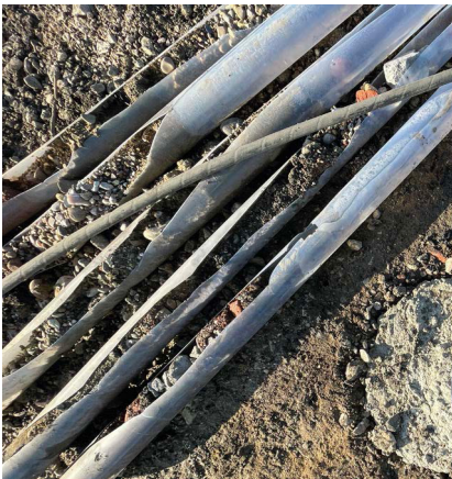
Additional site investigation helped target the in situ remedial design.
