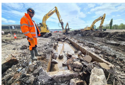
Soil remediation works being carried out by Vertase © Vertase FLI
