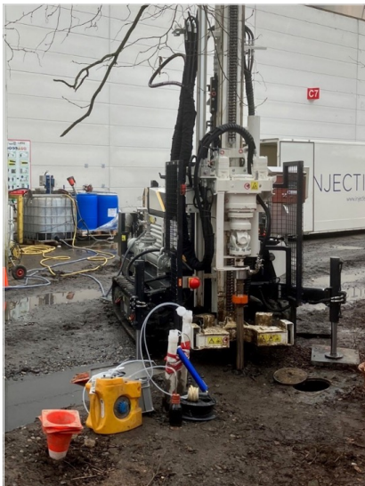
SourceStop is applied using the Spin Injector while samples are collected from monitoring wells to assess subsurface distribution.
