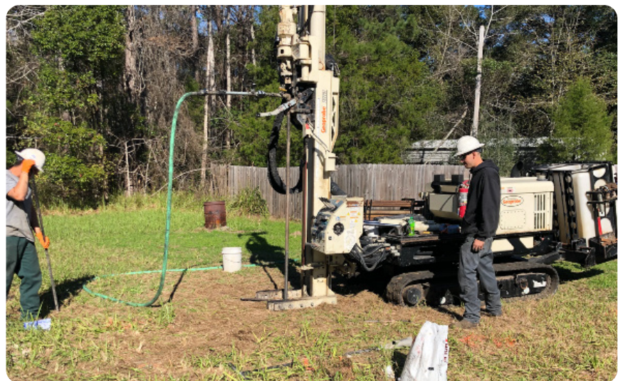
Injection of PetroFix using direct push injection methods
