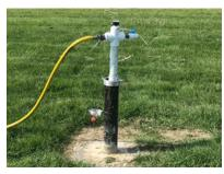
Example of an injection head assembly mounted to an above ground well.
