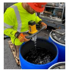
The image shows the homogenization of PetroFix using a high torque/high rpm mixer with appropriate mixing paddle.
