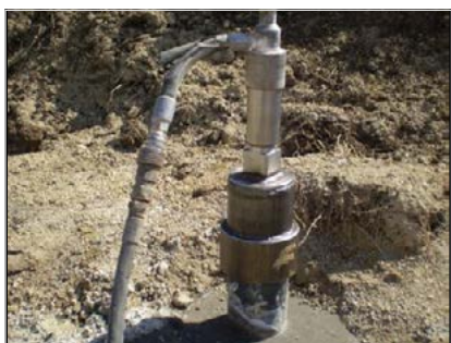
Pump outlet connected to well head
