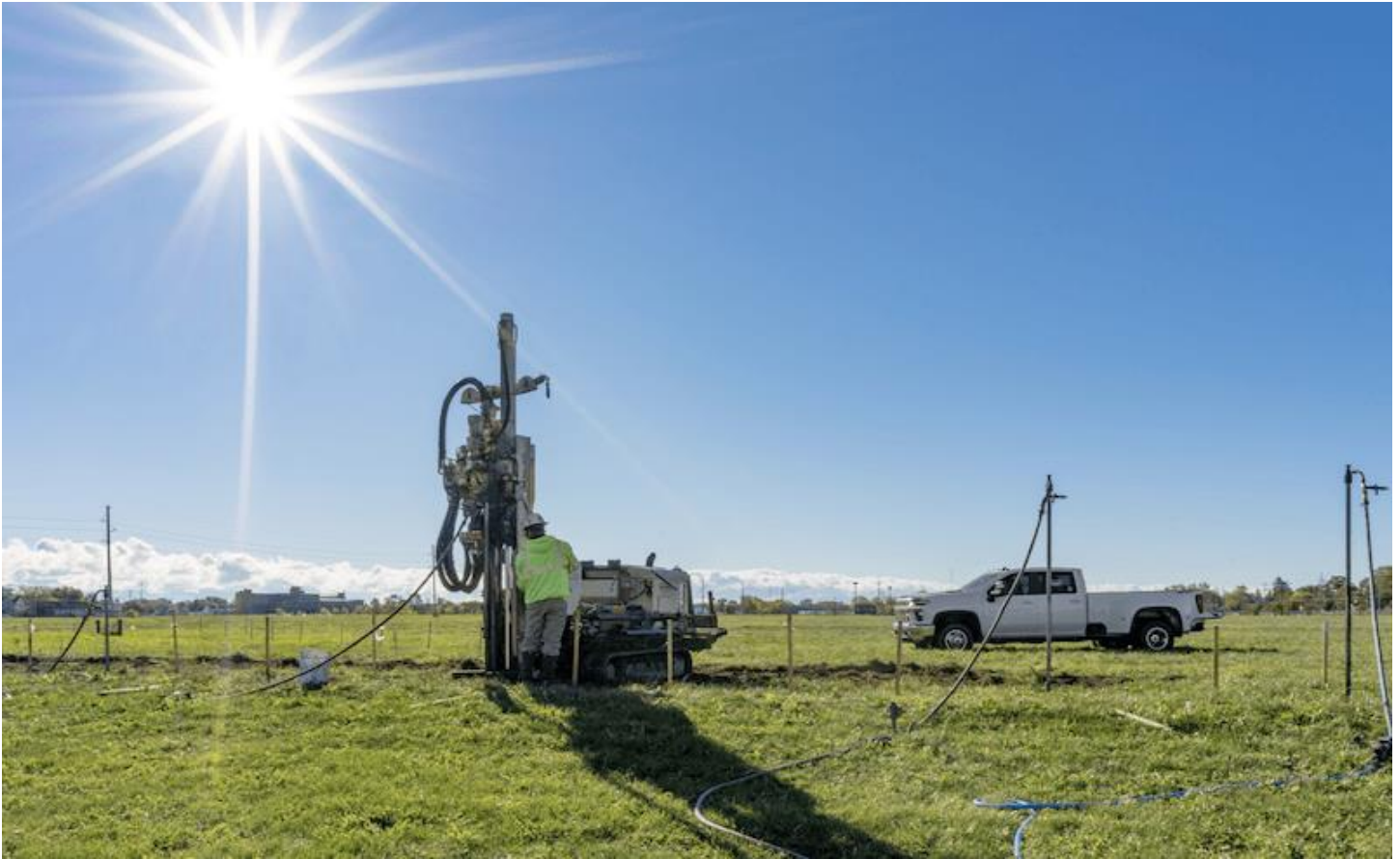
Field Injection of PlumeStop Colloidal Activated Carbon. (Photo credit: Angie McMonigal Photography LLC)
