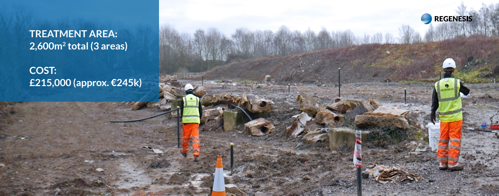
Fig.5 Full-scale treatment: Grid injection in source area 1
