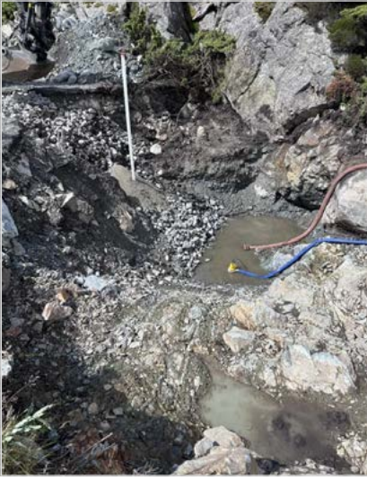
Excavation where the SourceStop barrier was implemented, shows crystalline bedrock geology.
