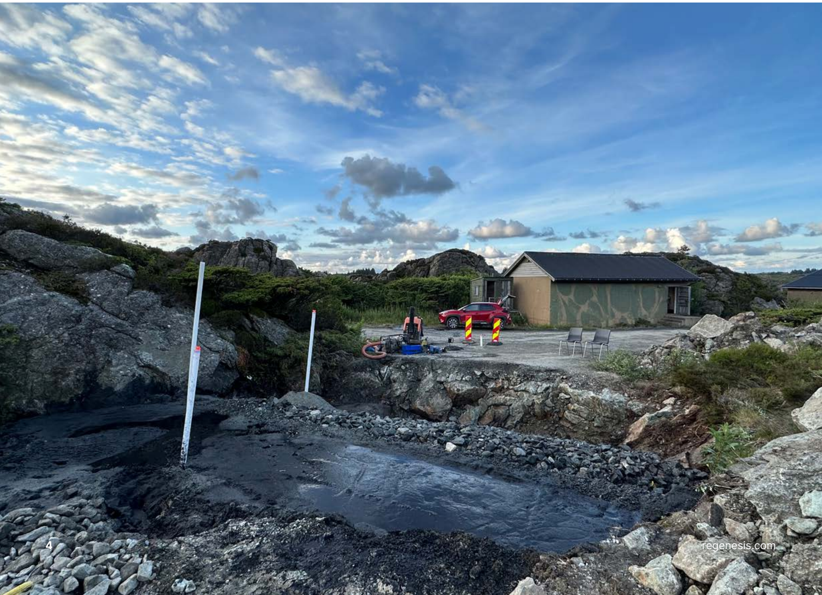
Excavation where the SourceStop barrier was implemented, shows crystalline bedrock geology.
