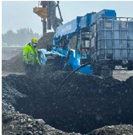
SourceStop spray-applied to NFS fill material
