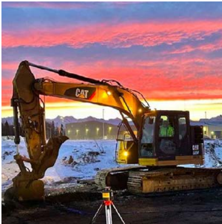
Excavation prior to installation of permeable trench barrier
