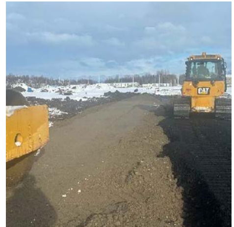
Placement of SourceStop-amended fill to create a permeable sorptive barrier
