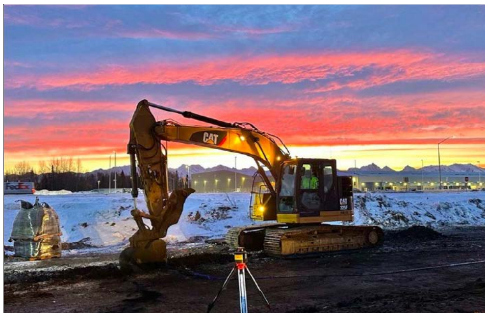
Excavation prior to installation of permeable trench barrier at Parcel 2
