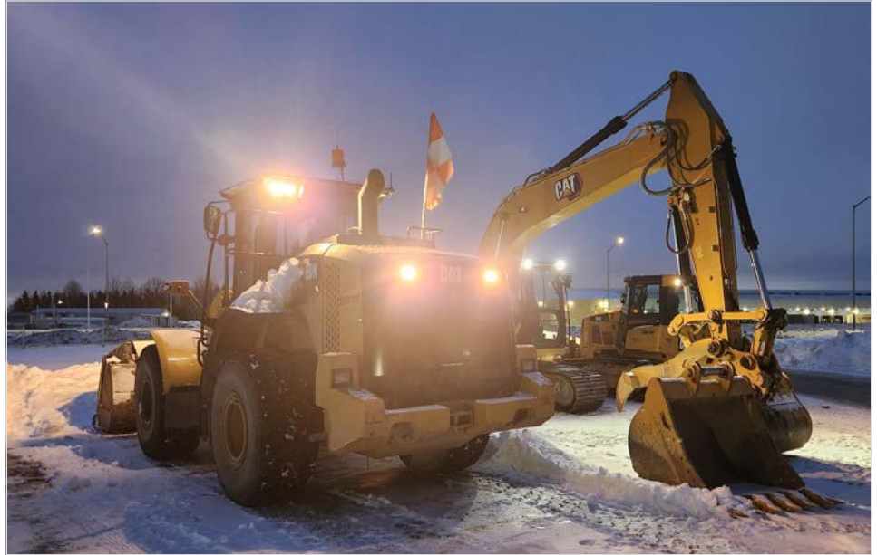
Winter Construction Schedule: Preparation and installation of the engineered fill and PFAS treatment zones.
