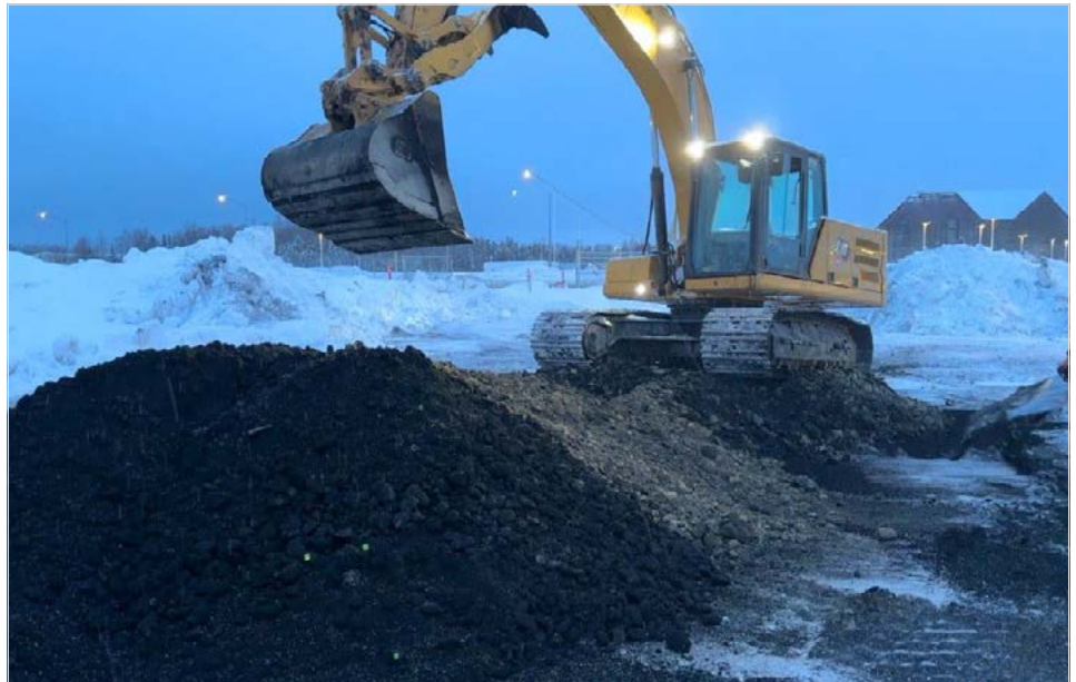
SourceStop is mixed into NFS fill material before placement into trench barrier.
