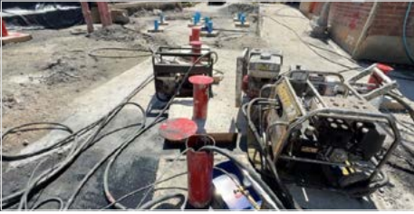
The injections took place into pre-installed wells
